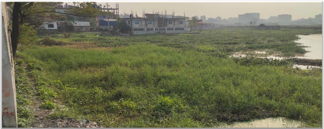
Figure 4.86: Matuail Uttar bondhe Field is spoiled by sewerage water, Ward No- 63
