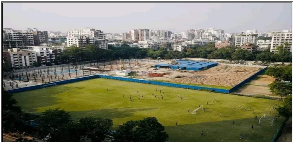
Figure 4.2: Abahony Club Field, ongoing construction for next sports complex
