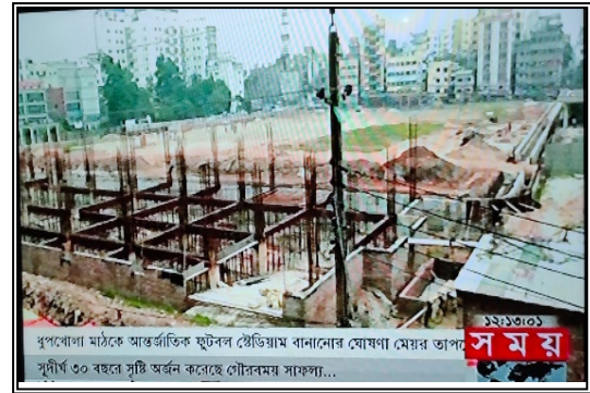
Figure 4.97: Ongoing Construction of Football Field in Dhupkhola,
