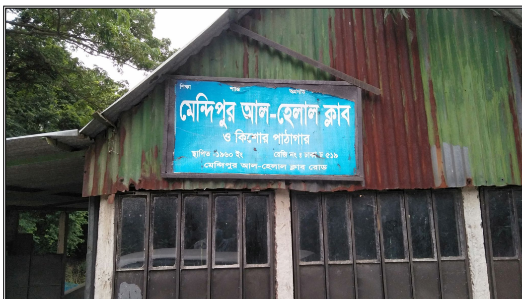
Figure 4.68: MendiPur Al - Helal Club Field, Ward No - 70. is drowned by flood water. In winter season, it will dry and it is open & free for all.
