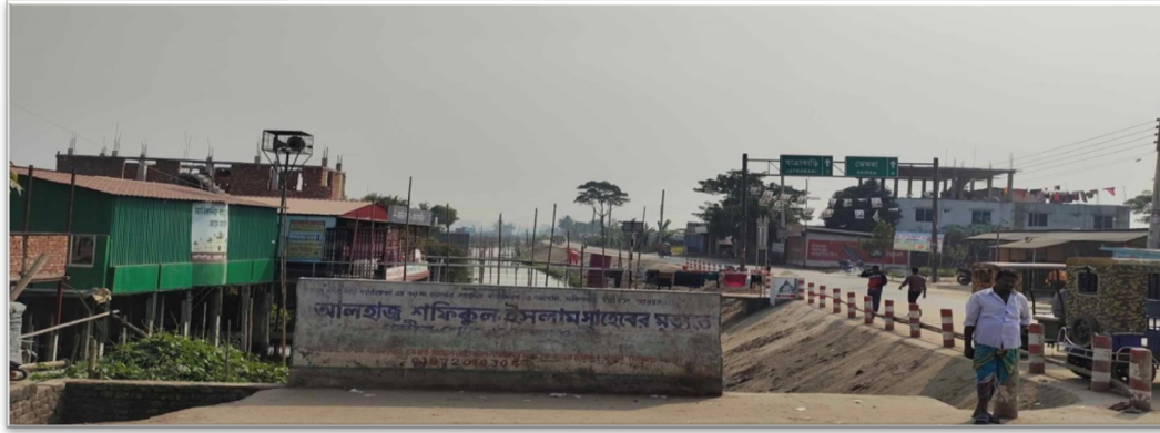
Figure 4.81: Huge large Khas (government) Land have taken possession in this canal, beside of WAPDA Road. Ward No- 73
