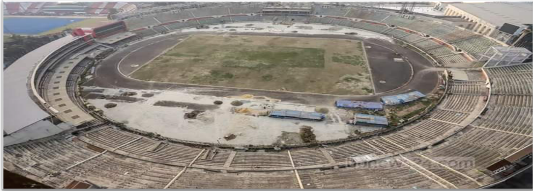
Figure 4.37: Bangabandhu National Stadium, Ongoing Reconstruction, Ward no – 13
